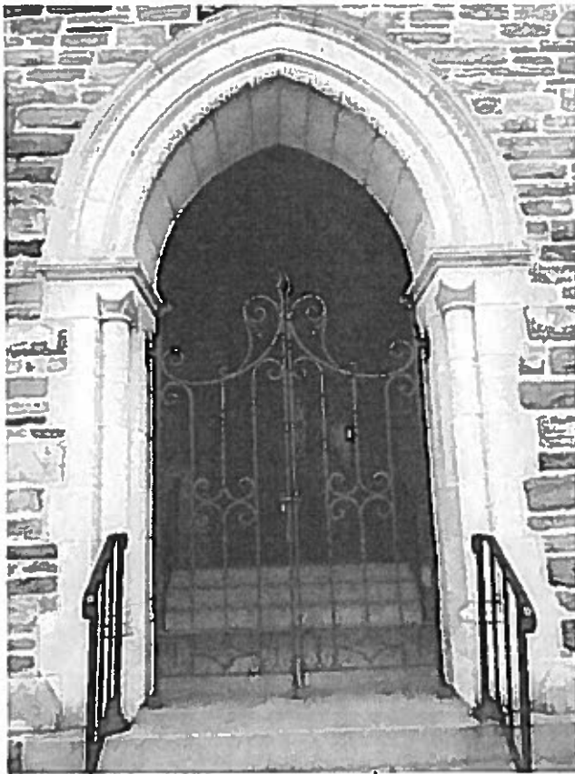
Image 6 – Detail of the entrance on 33 rd St.
