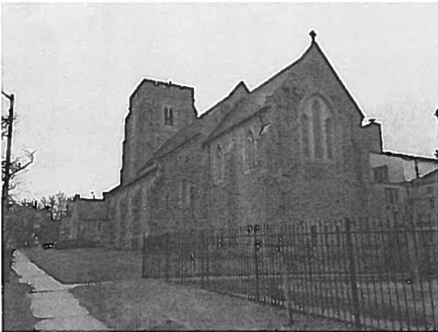
Image 5 – South elevation facing 33 rd St.
