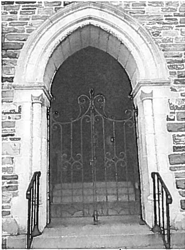
Image 6 – Detail of the entrance on 33 rd St.
