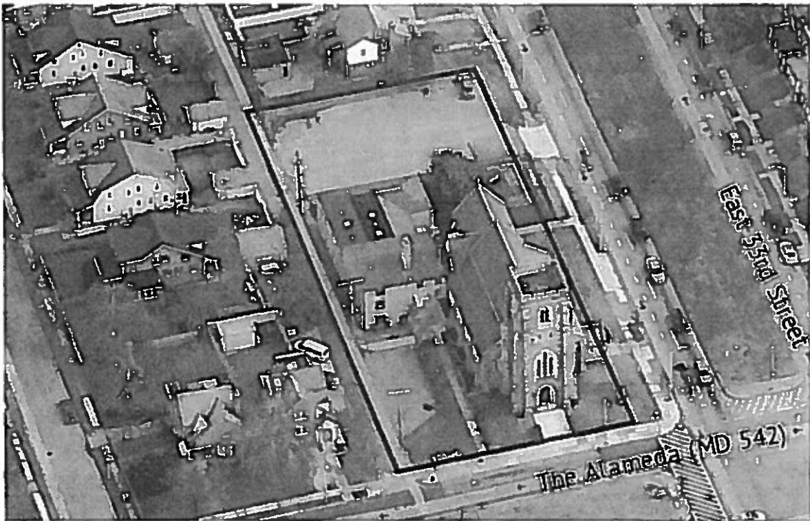
Image 1- Aerial view of site, view from northwest.
