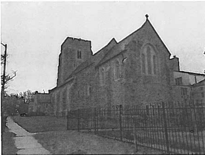
Image 5 – South elevation facing 33 rd St.
